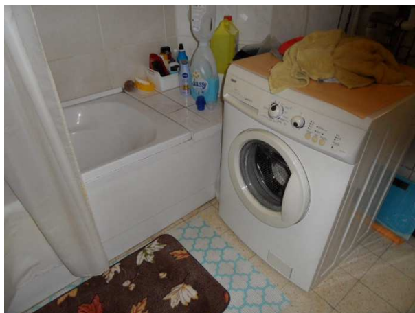
wasmachine in beschermingsvolume 2
